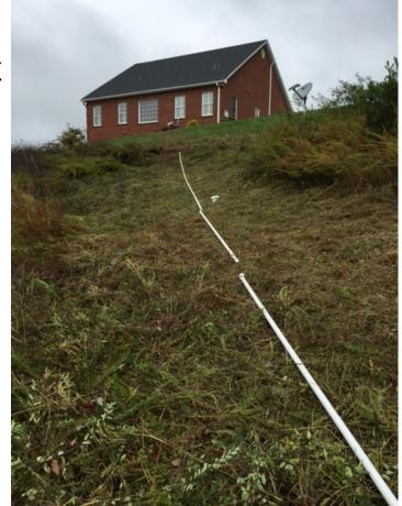
Found PL-259/SO-238 junctions using stud-finder, and then replaced connectors with soldered Amphenol. Of course, the short was at the last junction! 26
